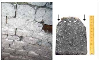
**Fig. 1:** Steel casting ladle with typical wear at the joints, "cobblestone formation", and open joints.
